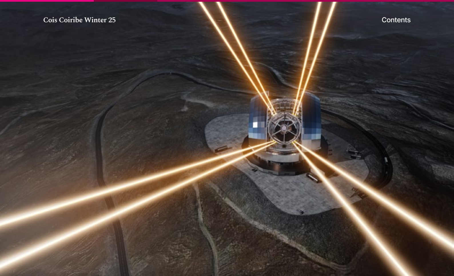
This artist's rendering shows a night view of the Extremely Large Telescope in operation on Cerro Armazones in northern Chile. The telescope is shown using lasers to create artificial stars high in the atmosphere. Credit: ESO/L. Calçada.
