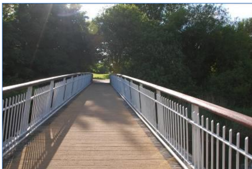
Plate 3 Pedestrian bridge, from s.
