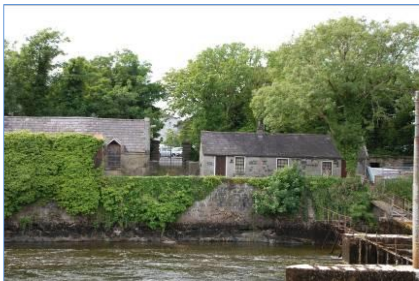
Plate 18 Site 9 Fisheries House, from se.
