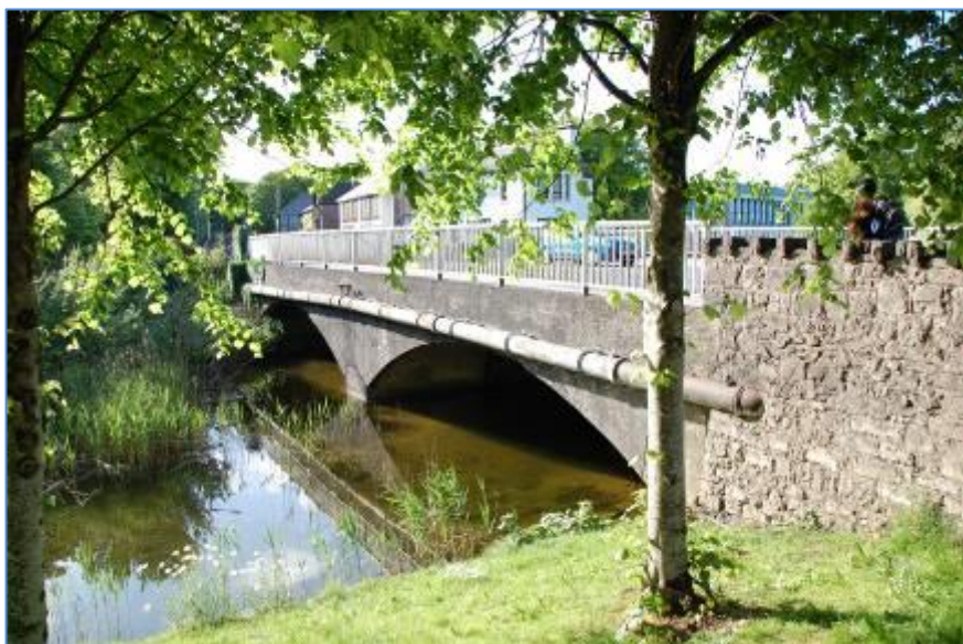
Plate 2 Beggars Bridge, from sw.
