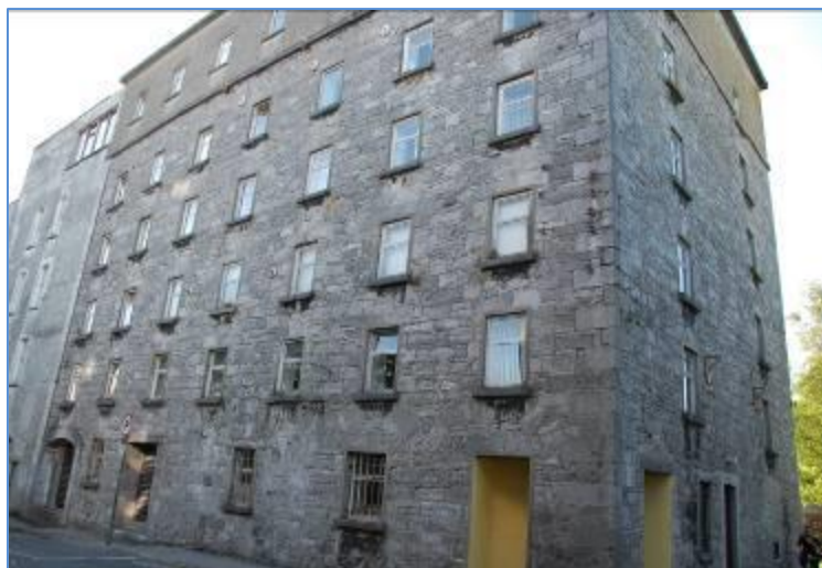
Plate 7 Hydrology Department, from se.
