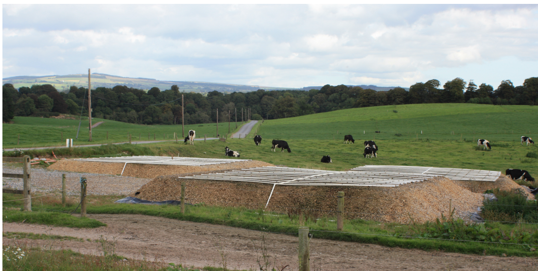
Figure 4.1 Overview of the three farm-scale filters, as constructed
