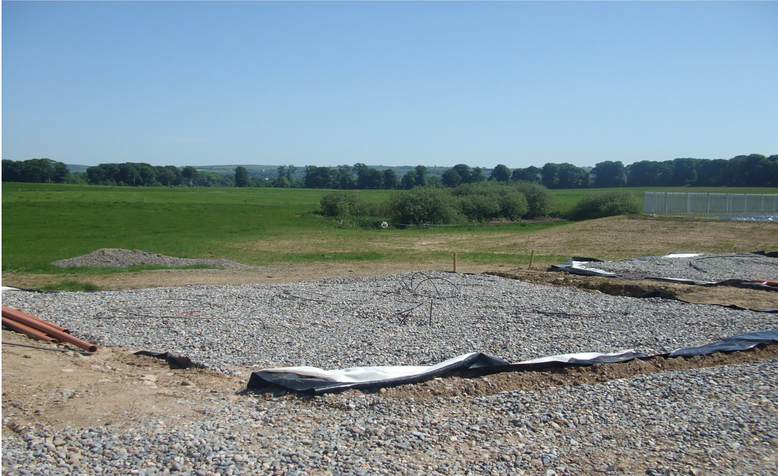
Stone layer creating a level base for the woodchip
