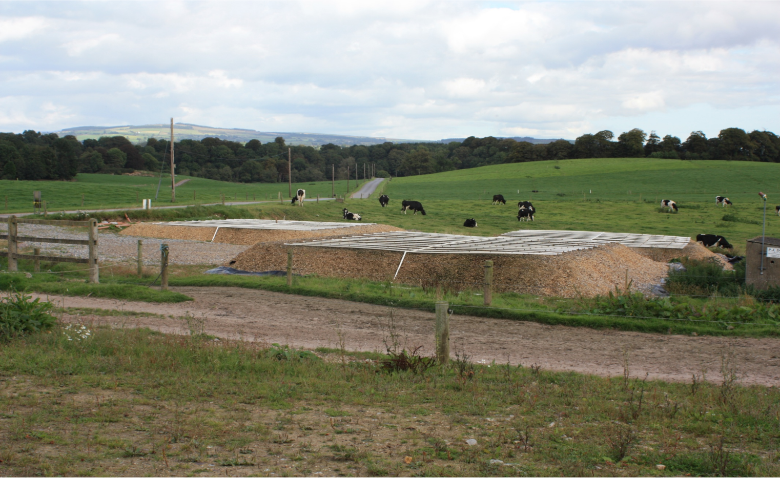
Overview of the three-replicate farm filters with the distribution system on top
