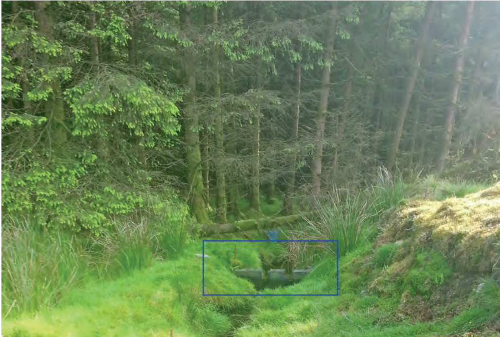
Figure 2.13. Downstream silt trap (within blue box) at Kilcoagh site (photograph: John Clarke, UCD).
