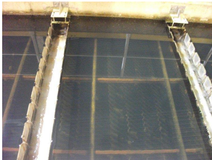
Figure 2.4 A sedimentation basin with angled lamella.
