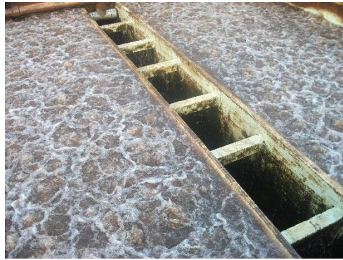
Figure 2.6 Backwashing of a rapid gravity filter.
