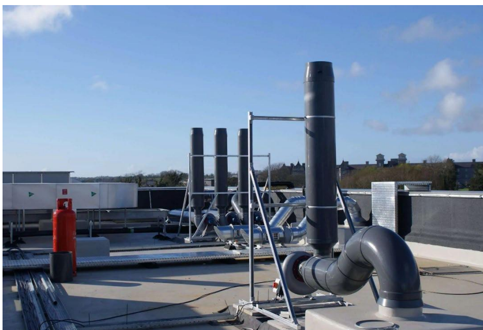
Image 3: External extract fan and ducting roof mounted.
