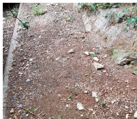
Figure 17 Earth bank located in the North of the campus
