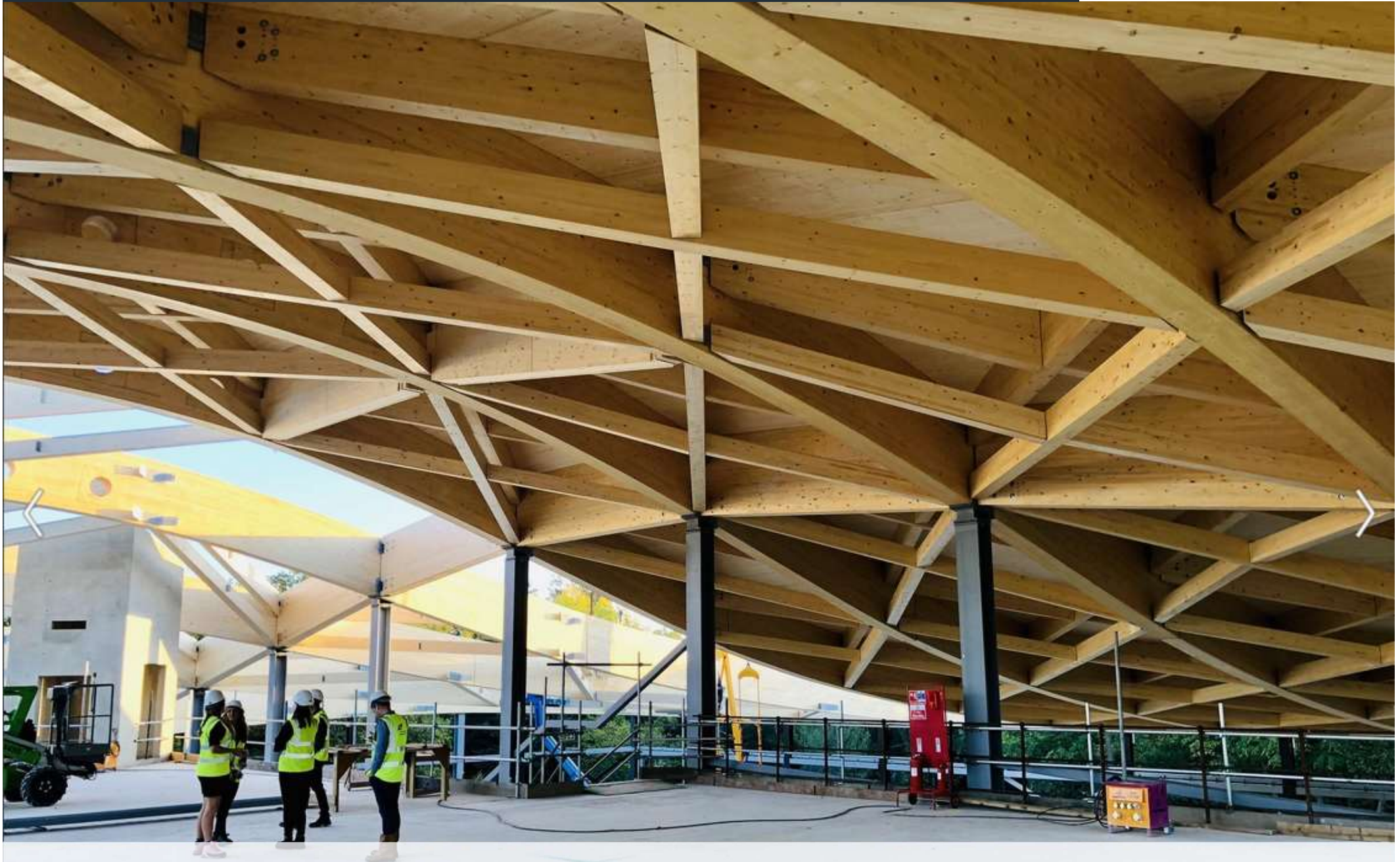
Sportshall, Complex 3D roof shape, diagonal double layer purlins, CLT roof deck, parametric design
