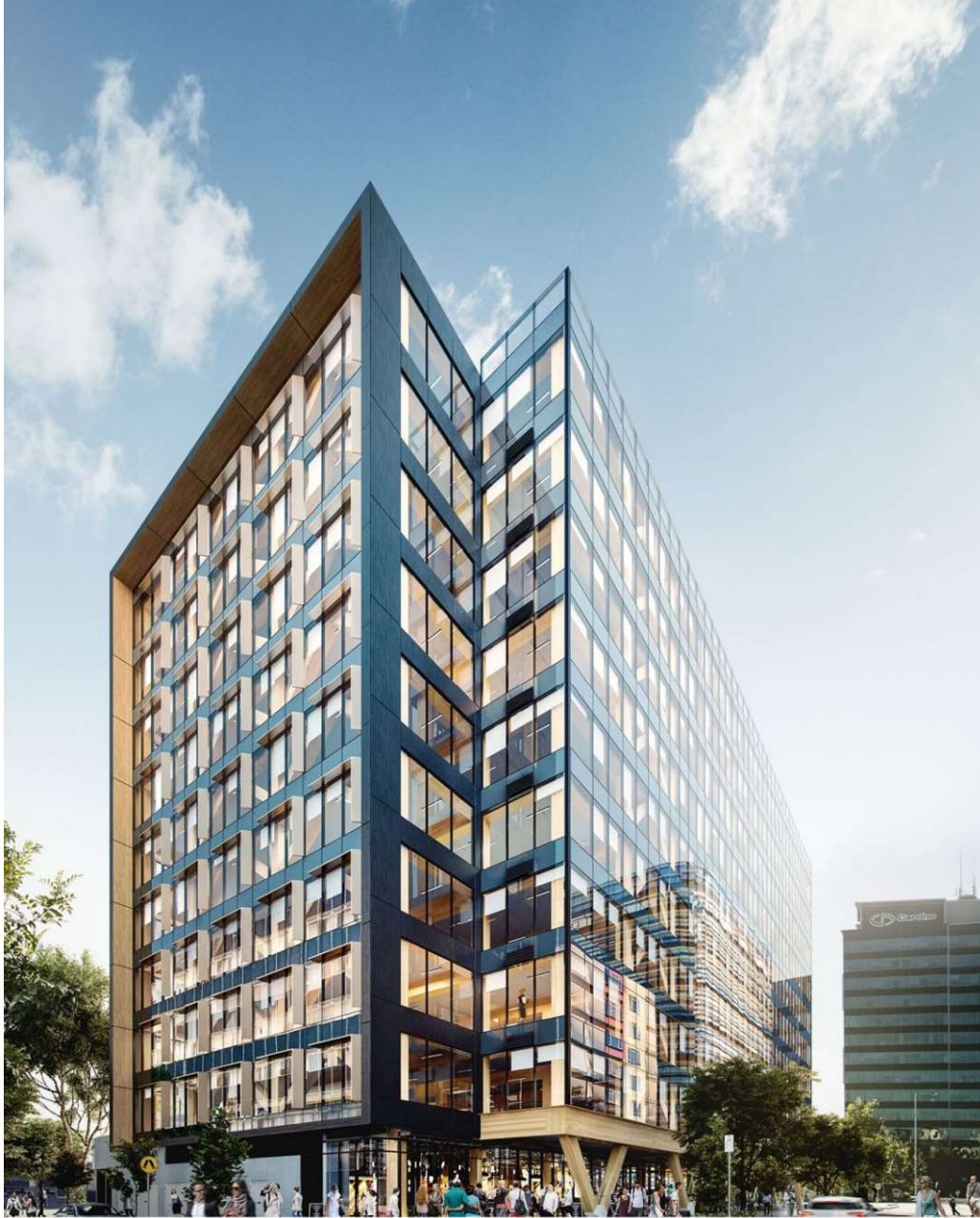
52m high, largest engineered timber office block in the world, Glulam kit by Wiehag
