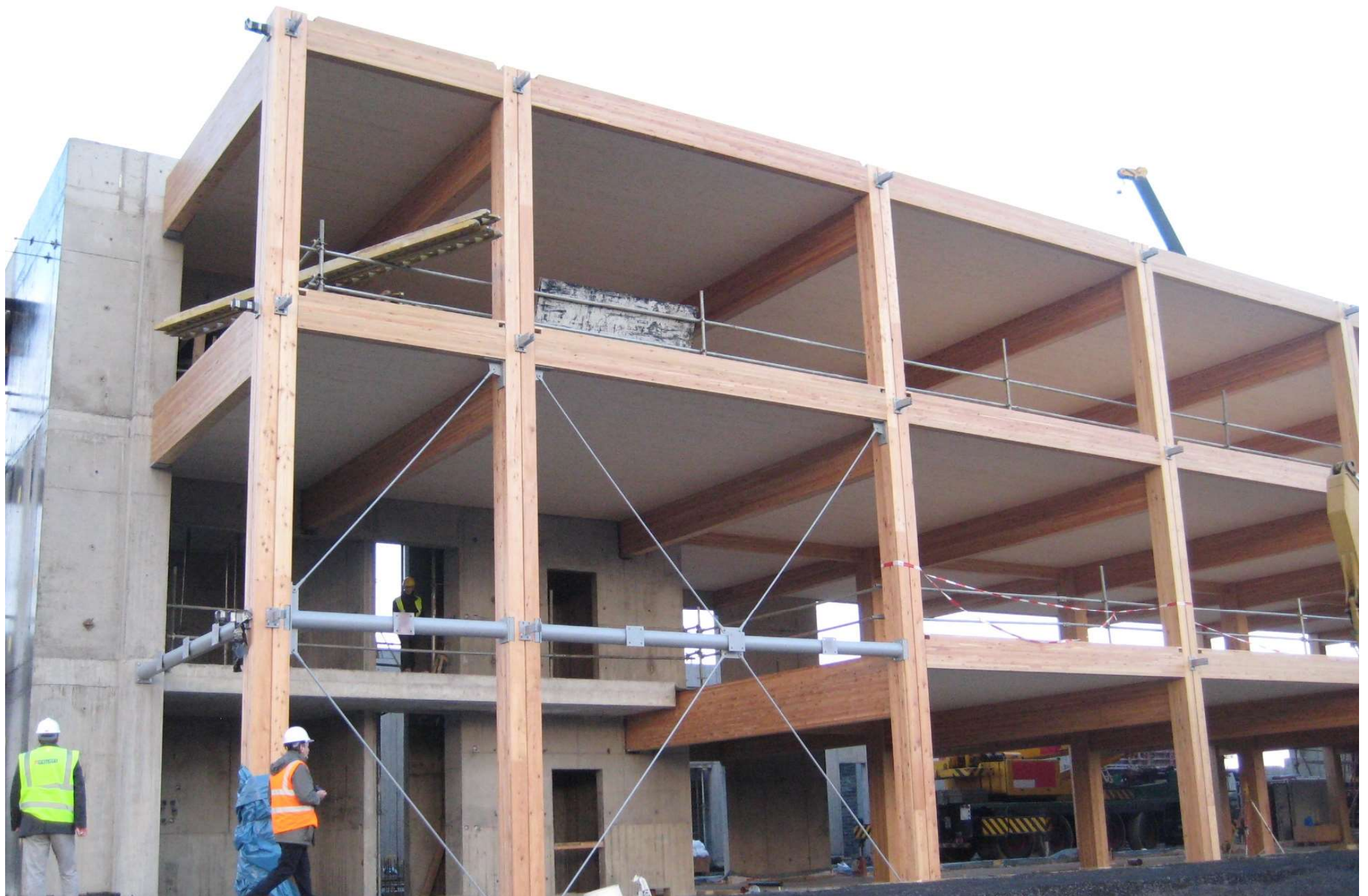
Office Building Ballyogan, IRE
