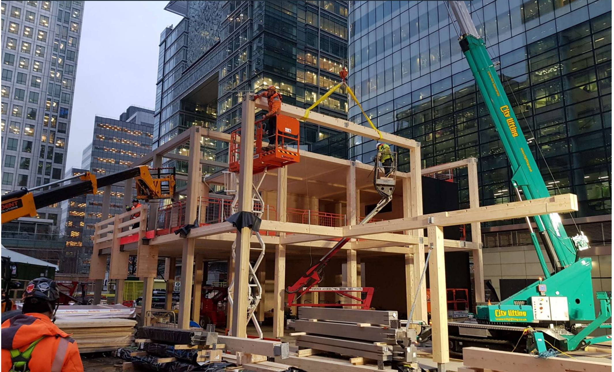
Glulam structure and CLT slabs, walls Exposed timber in Accoya
