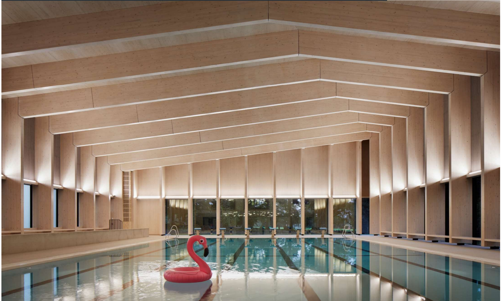
Glulam portal frames, CLT on roof and walls, white wash
