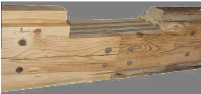
Fig. 6. Shear reinforcement with GFRP.
