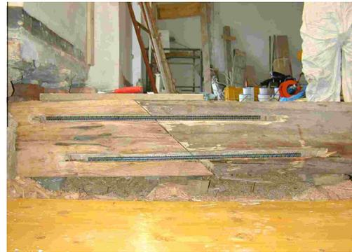
**Fig. 4.** Linking grooves.
