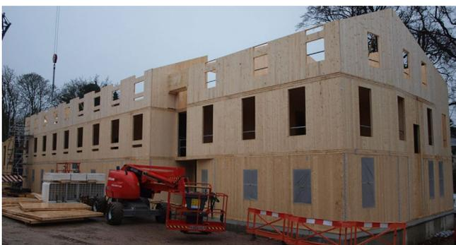
Figure 3. Platform construction [Image: C UíChúláin].
