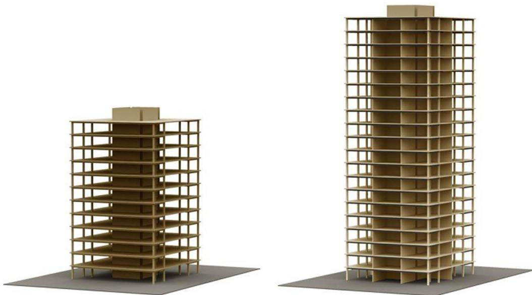
Figure 12. FFTT building frames: Options 1 (12-storey) & 2 (20-storey) (Green, 2012).
